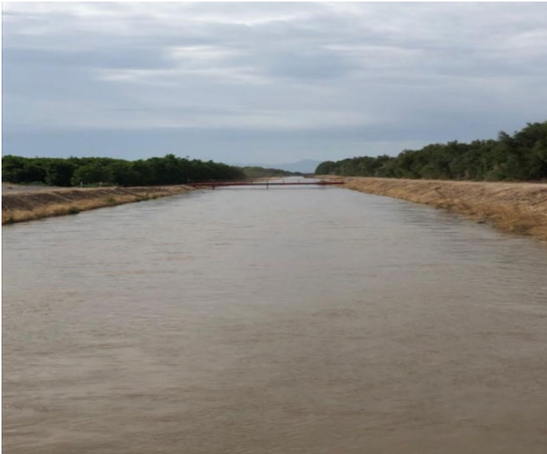
Lateral, Mesilla Valley June 2022
